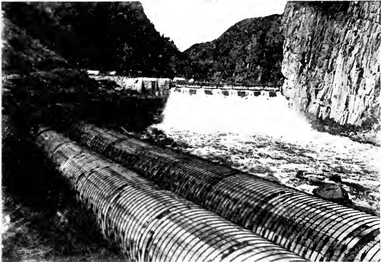
FIG. 68.—Montana Power Company. Dam and Wooden Penstocks for Madison No. 2 Plant.
